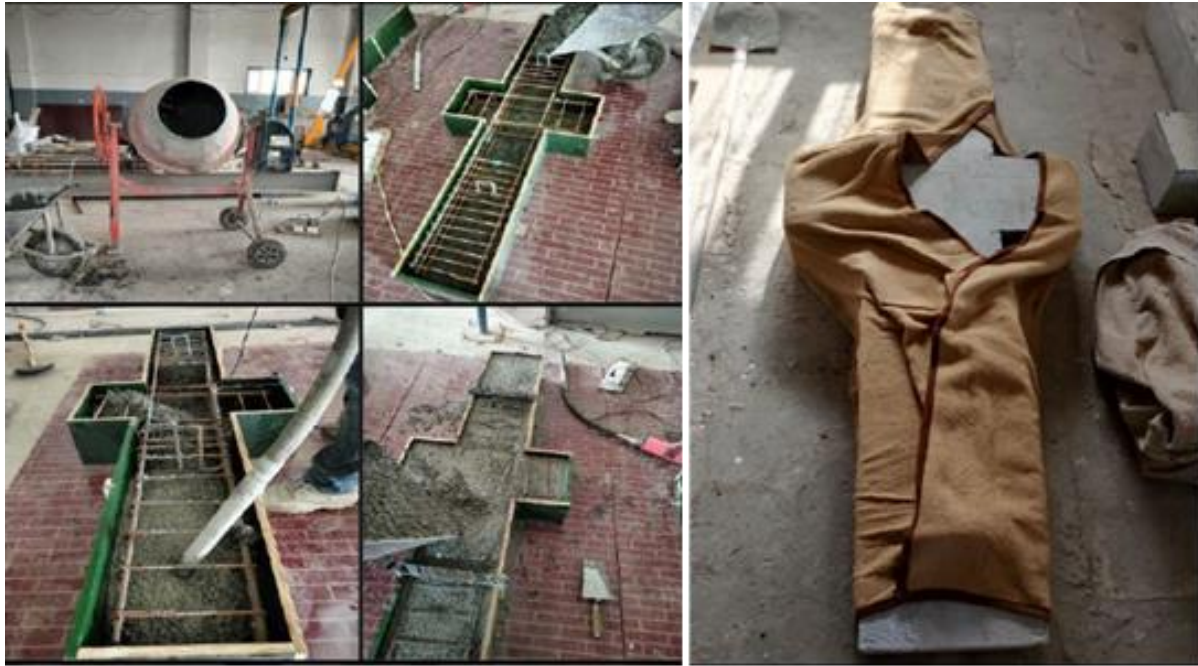
Casting of beams with mixture.
