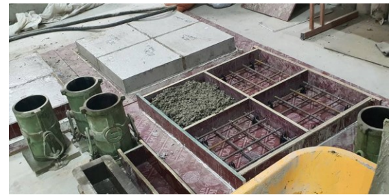
(a) Slab Shuttering and Reinforcement.
