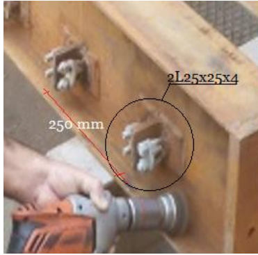
Fig. 7 Location of Double Angle (2L25x25x4).
