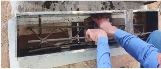
Fig. 5 Reinforcement of Steel.
