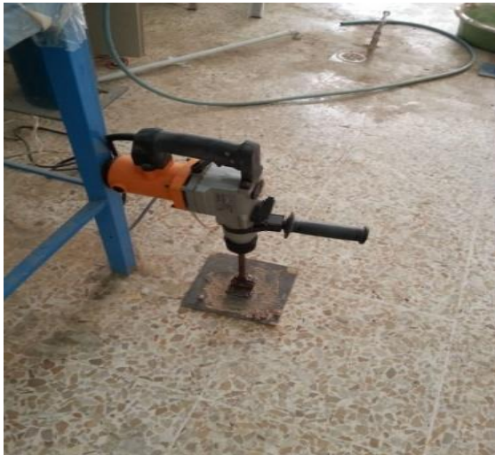
Fig. 4 Electrical Compactor Used.
