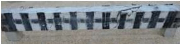
Figure(7)Crack pattern at failure for beam B2.
