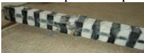
Figure (9)Crack pattern at failure for beam B3.
