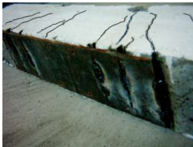
Figure. (17) View of Cracking of Beam B15 (100% preloading, debonding in one welding point )
