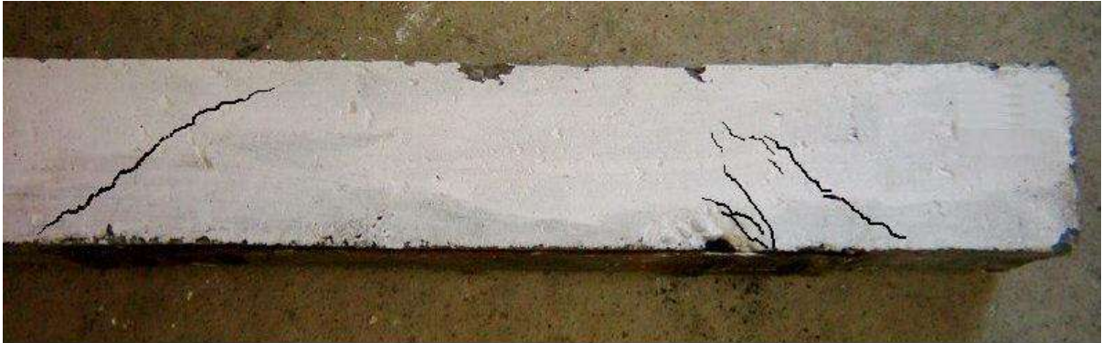
Figure. (15) View of Cracking of Beam B12 (No preloading, No debonding occurs)
